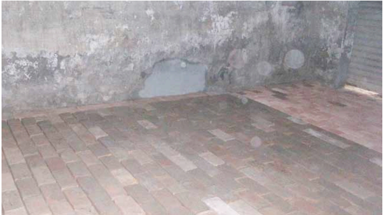
Floor of principal office.
