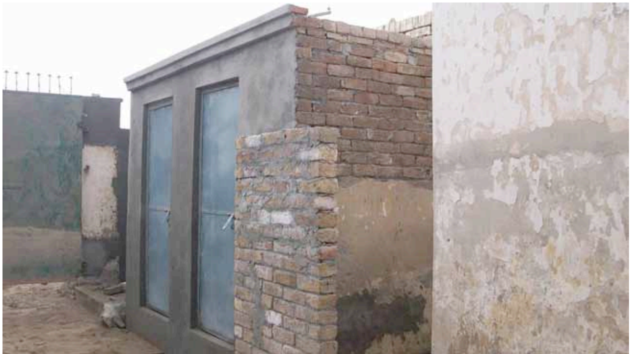
New construction of two washrooms
