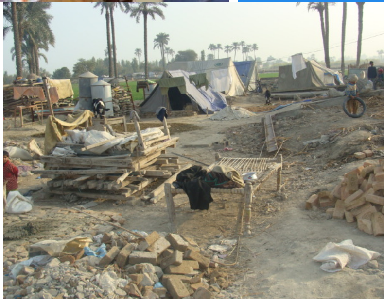
Scene of demolished houses and debris.
