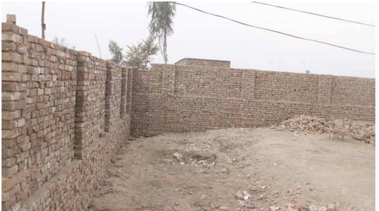
Boundry wall after construction
