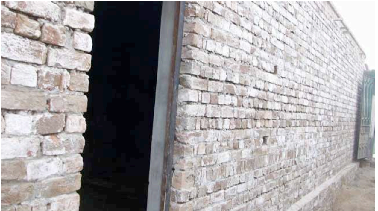
Outer wall of principal office after construction
