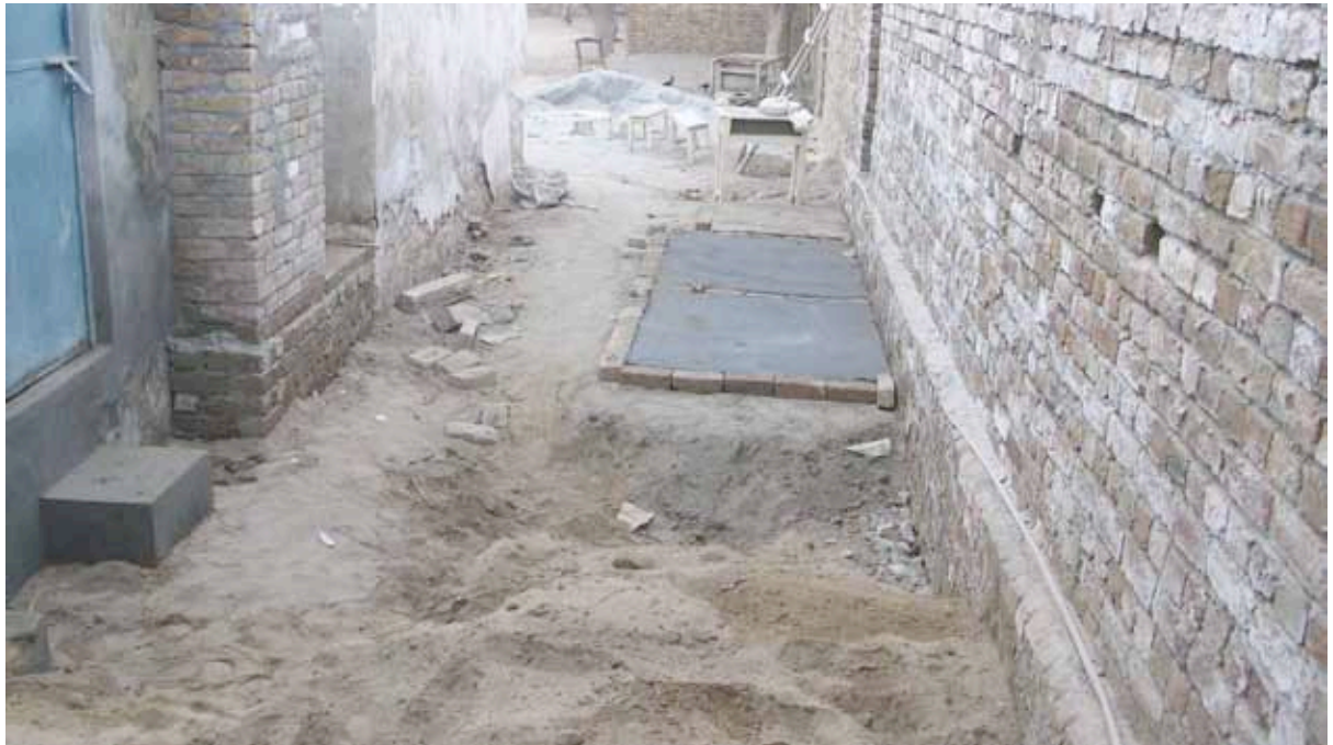
Two main holes after construction
