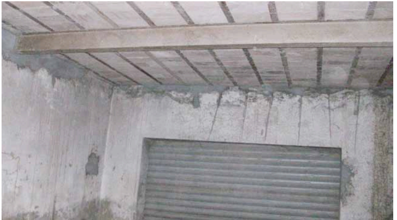
Principal office roof after repair
