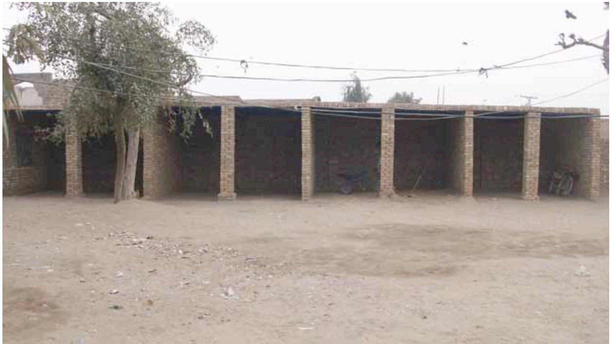
Four classrooms after construction in replacement of shades
